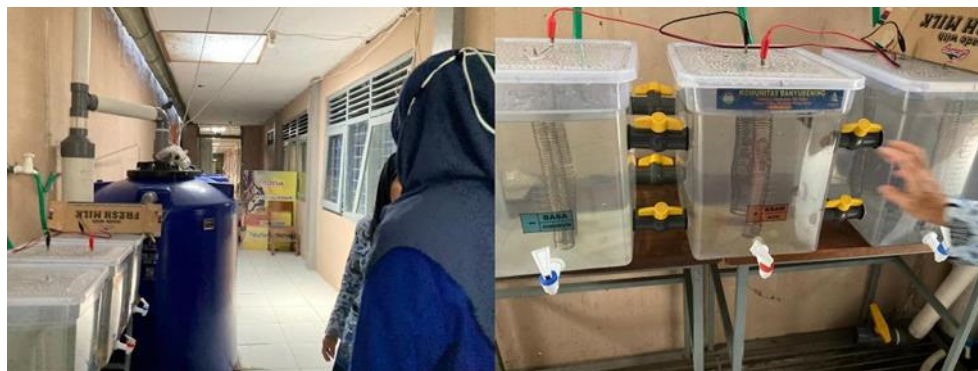
Gambar 1. Instalasi Rain Water Harvesting
